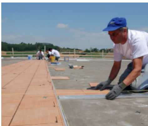
Laying ceramic tiles with Kerabond + Isolastic
