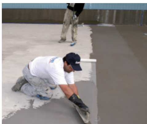
Waterproofing a swimming pool with Mapelastic Zero
