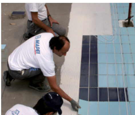
Application of ceramic coating on Mapelastic Zero
